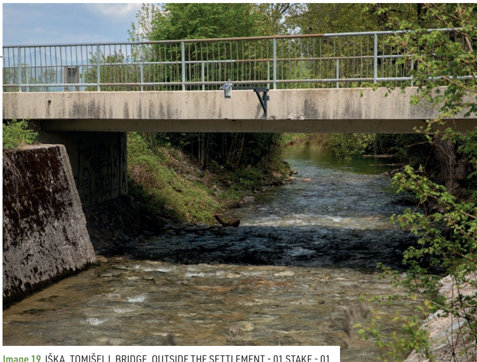
Image 19 IŠKA, TOMIŠELJ, BRIDGE, OUTSIDE THE SETTLEMENT - 01 STAKE - 01
