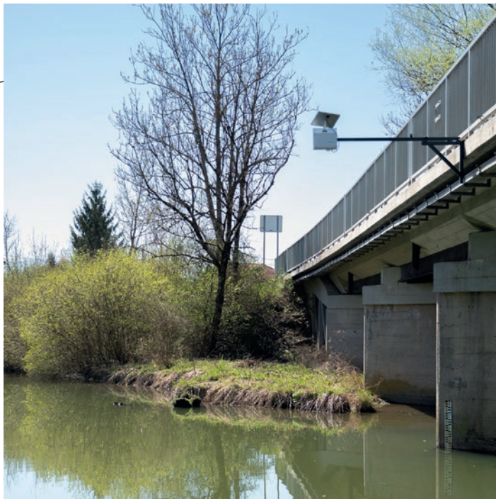
Image 27 IŽICA, BRIDGE ON IŽANSKA ROAD, KAROLINKA, BRIDGE - 01
