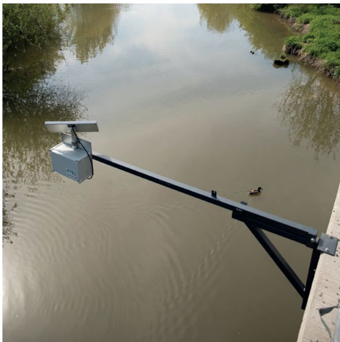
Image 28 IŽICA, BRIDGE ON IŽANSKA ROAD, KAROLINKA, BRIDGE - 02
