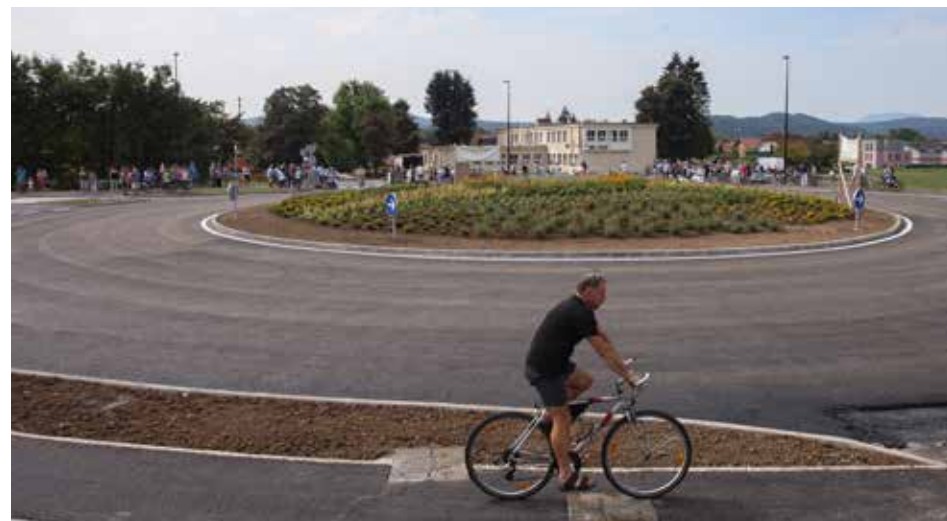
We renovated the road Zaloška cesta, built a roundabout, constructed sidewalks and bicycle lanes on both sides, set up an LPP bus stop... Construction of bicycle lanes and pedestrian surfaces falls under the scope of the cycling network development project of the City of Ljubljana, which is partly co-financed by the EU Cohesion Fund and the Republic of Slovenia. Photo: Nik Rovar
