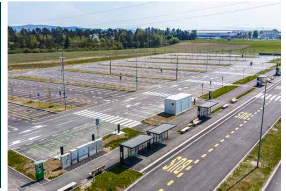
The new, already sixth P+R parking area has 392 parking spaces, including spaces for the disabled, electric cars, buses, tourist buses and 15 parking spaces for caravans. There are also 20 bicycle stands under a roof with space for 40 bicycles at a time, and 100 bicycle stands without a roof for 200 bicycles at a time. From those, the first 12 stands are equipped with chargers for 24 electric bicycles, and there are 16 bicycle storage lockers with chargers for electric bikes. The new parking area P+R Stanežiče is, like all others, connected to the city centre with an LPP bus line. Photo: Doris Kordić
