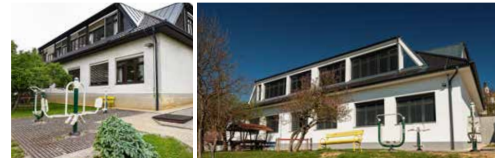
BEFORE The Oskar Kovačič Primary School building, Rudnik subsidiary, before the renovation. NOW The Oskar Kovačič Primary School building, Rudnik subsidiary, has undergone a comprehensive energy renovation. Photo: Peter Irman
