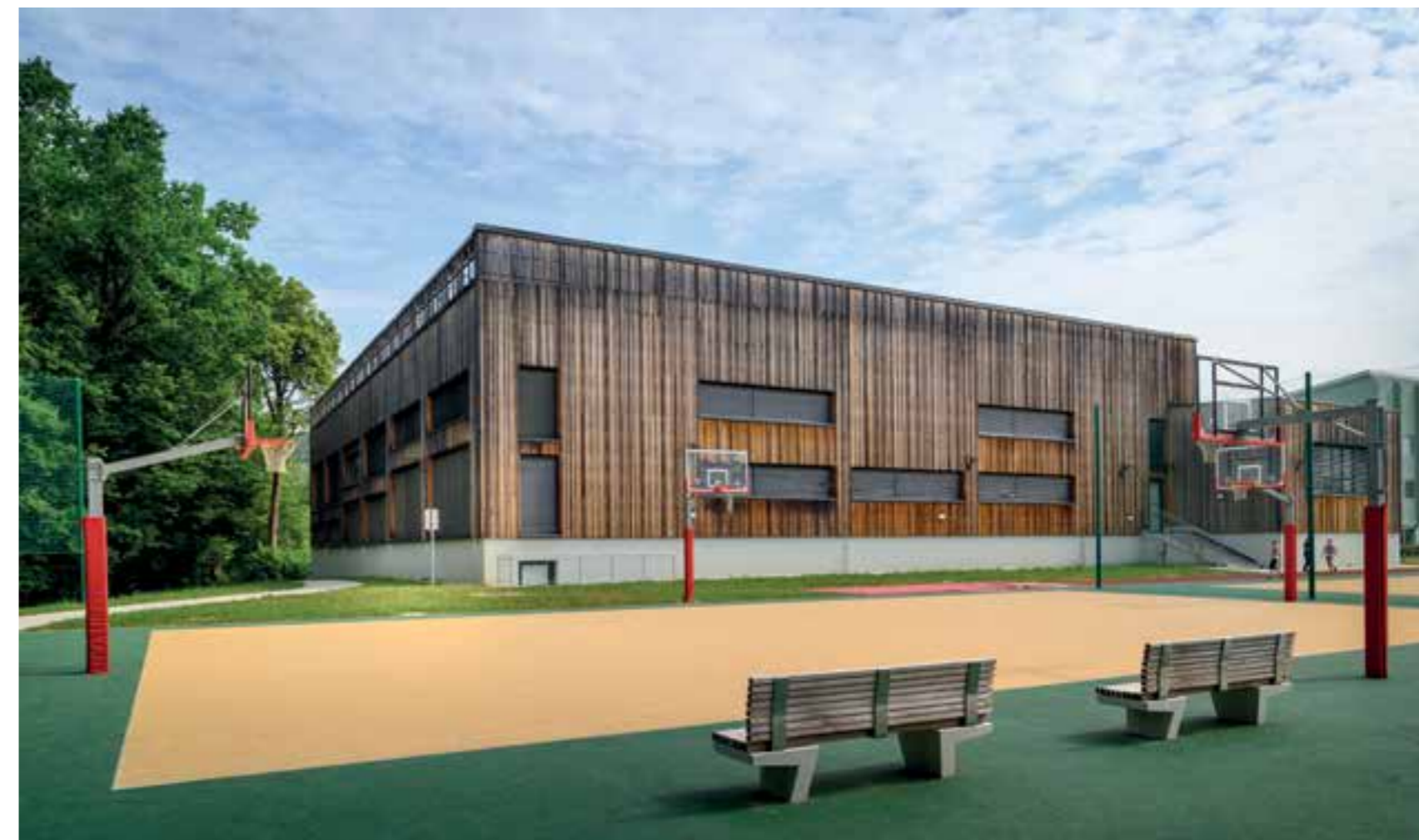
The National Hero Maks Pečar Primary School has a new gym, outdoor school, and recreation playground and is fully renovated.
