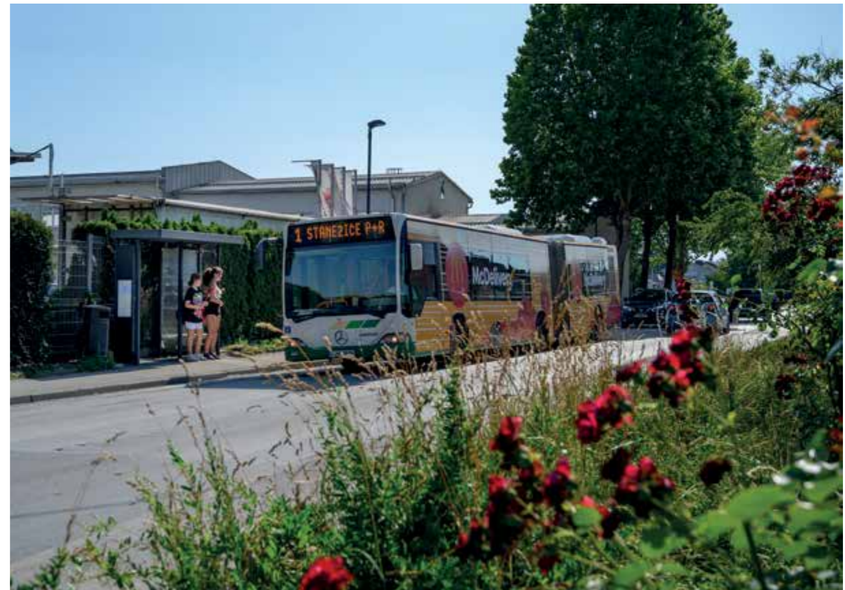
The new canopy at the bus stop of line 1 was arranged as part of the small works project.
