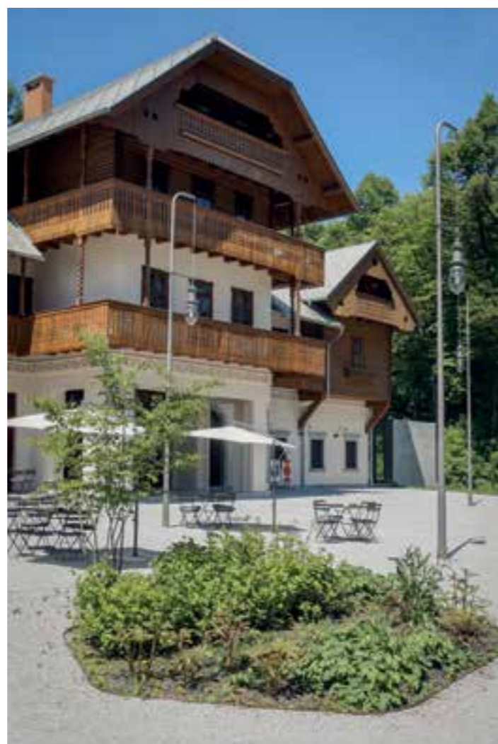
Before the renovation, Švicarija (The Swiss House) was overgrown, abandoned, and overbuilt, and some of its sections were damp and on the verge of collapse. Today, this completely renovated building in the heart of nature is a modern art centre with studios, artists' residences, and space for exhibitions, events, and educational programmes.
