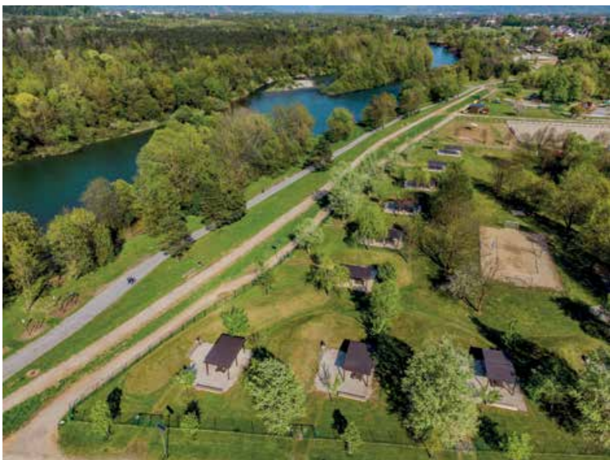
The refreshed image of the city is evidenced by the many renovated areas that used to be degraded areas, illegal landfills, or illegal small gardens. This is also the path directly along the Sava river, a total of more than 80 hectares of land for quality leisure time and relaxation in nature.
