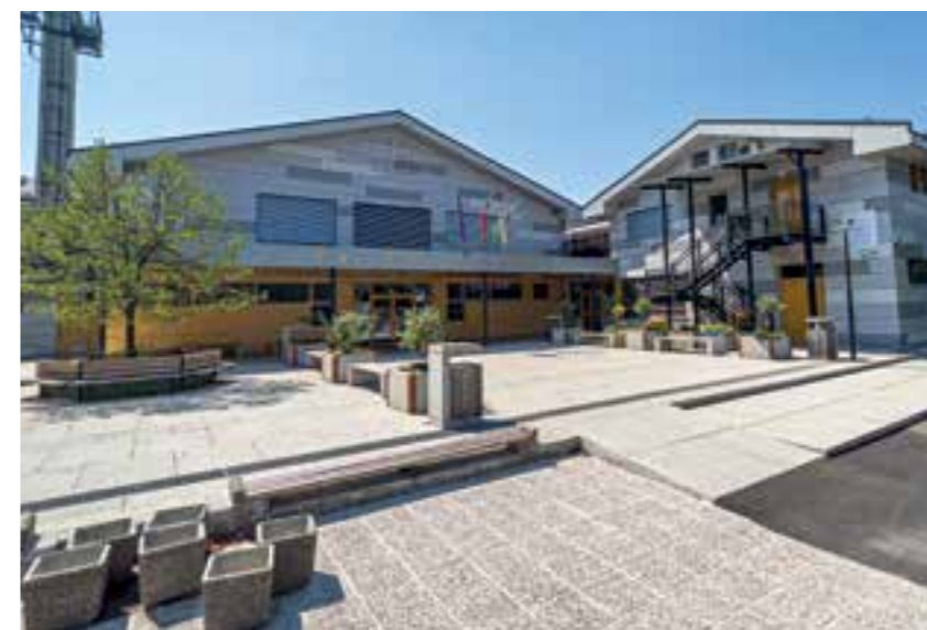
We added two new classrooms to the Livada Primary School.
