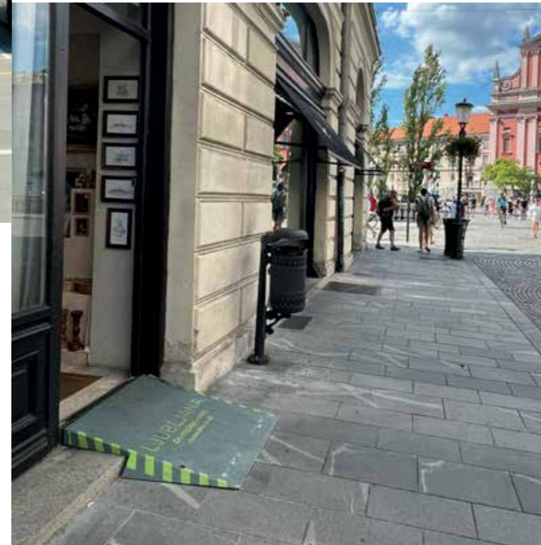
By installing ramps, which are entirely made in the wooden workshop of the Voka Snaga public company, we facilitate access to the city-owned premises in the old city centre, and at the same time we also encourage private owners of shops and bars to follow the city's example and adapt the entrances to their buildings as well.
