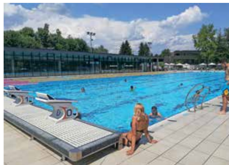
In 2015, we completely renovated Kolezija, the dilapidated and non-functioning Ljubljana swimming pool, and dedicated it to sports, recreation, and socialising.
