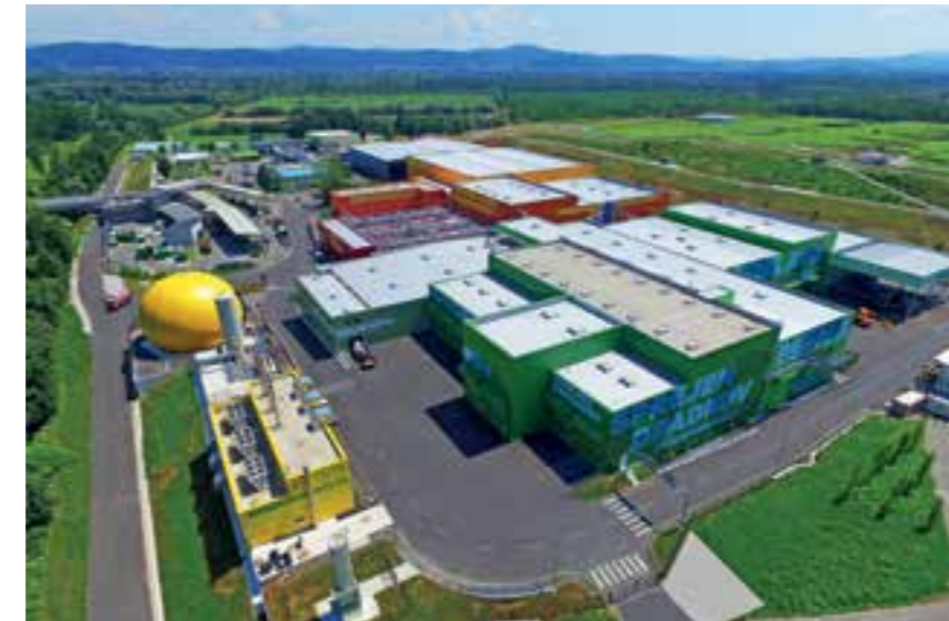
In 2015, the Ljubljana Regional Center for Waste Management (RCERO Ljubljana); a new, state-of-the-art facility for sustainable waste processing, became an exceptional asset for the city.
