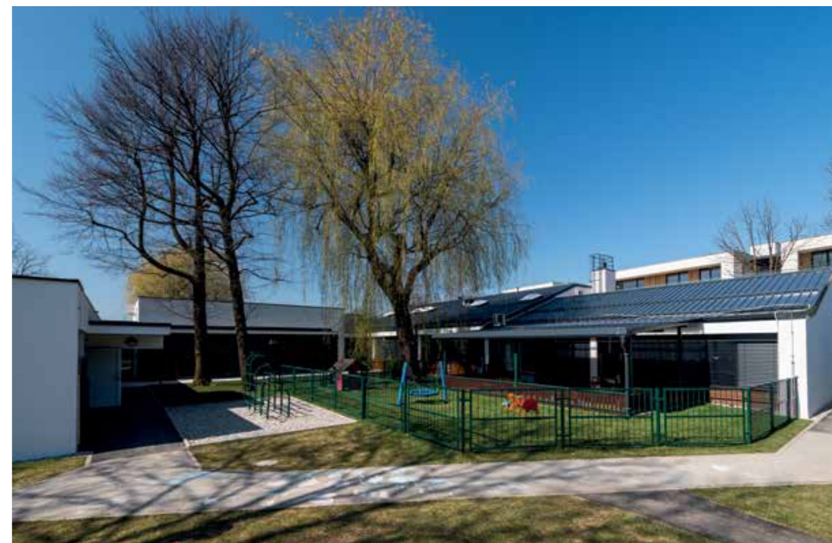
Fully renovated kindergarten Kolezija, Murgle unit
