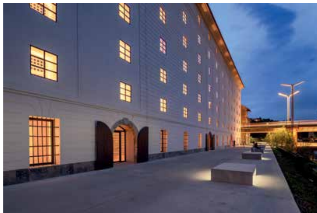
The comprehensive renovation of the Cukrarna Gallery was co-financed by the European Regional Development Fund and the Republic of Slovenia.
