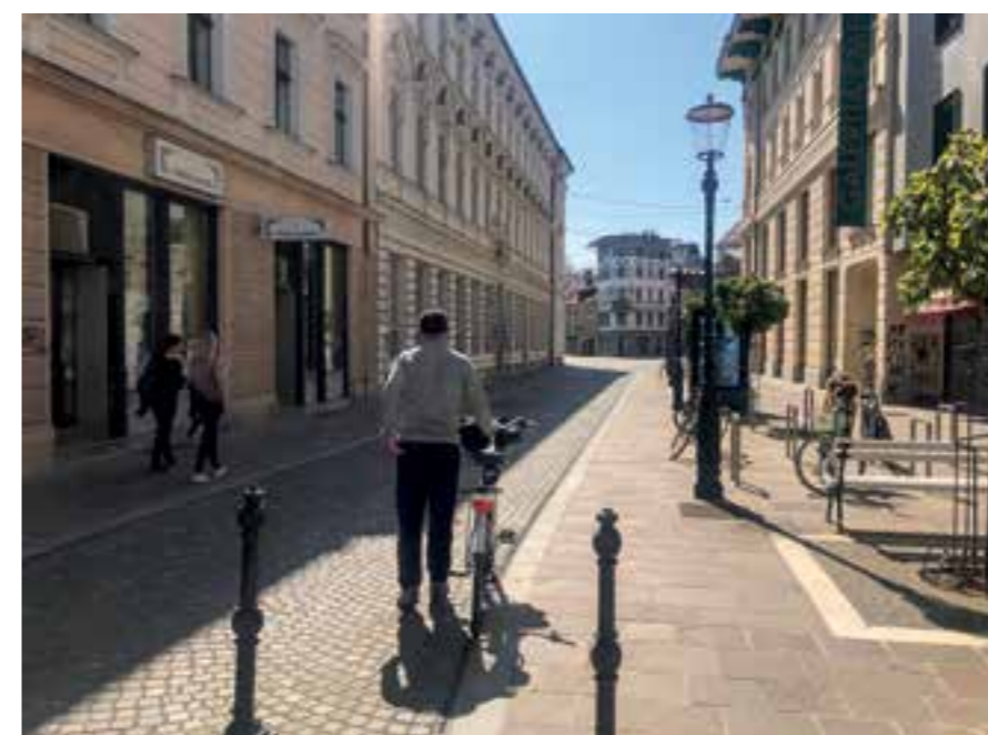
In addition to the new look, the comprehensive renovation of Trubarjeva cesta also included the renovation and construction of sewerage, water supply, gas supply, heating supply, optical fibre infrastructure and public lighting. As part of the renovation, we also renovated the connecting streets, namely Obrežna steza, Za čreslom and Prečna, Kastelčeva, Znamenjska, Usnjarska and Vidovdanska ulica. The European Union's Cohesion Fund and the Republic of Slovenia partially co-financed the project.
