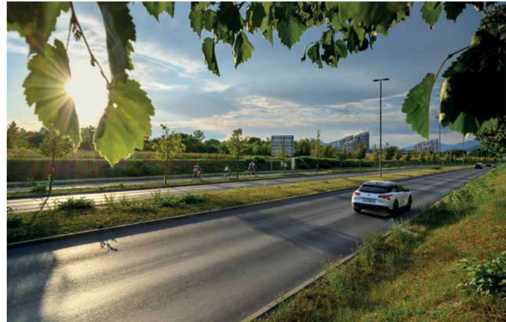
Many streets and roads have been renovated or rebuilt. In 2010, among others, we completed the construction of Štajerska cesta from the Tomačevo roundabout to the Žale roundabout, which shortened distances and brought many parts of the city closer together. Perhaps not so visible at first glance, but extremely important for the quality of life, is the newly built utility infrastructure in many parts of the city.
