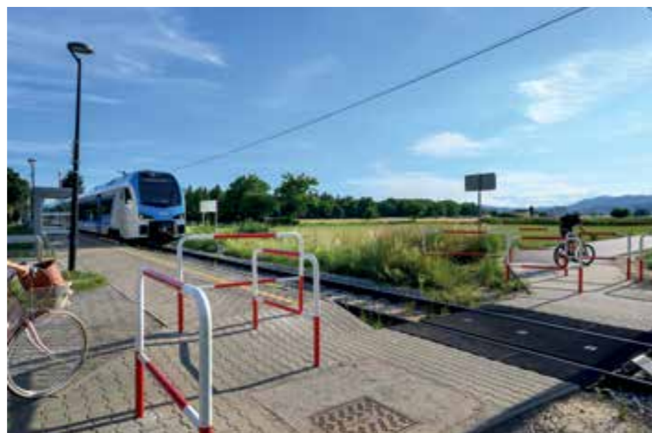
The level crossing over the Ljubljana Ježica railway track is finally safe.
