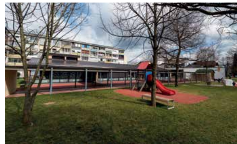
The fully renovated kindergarten Miškolin, Rjava cesta unit
