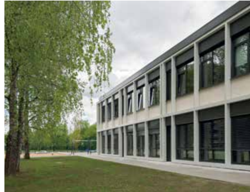
New extension, playground and comprehensive renovation at the Martin Krpan Primary School
