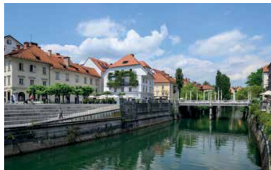
A view of the Jurčičev trg and the restored building »Zlata ladjica«
