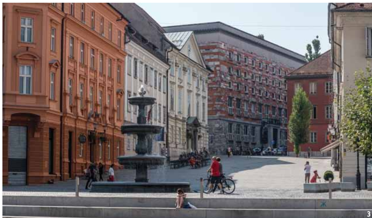
3 Narodna in univerzitetna knjižnica, pogled na palačo z Novega trga (foto: B. Zupančič). National and University Library, seen from New Square (photo: B. Zupančič).
