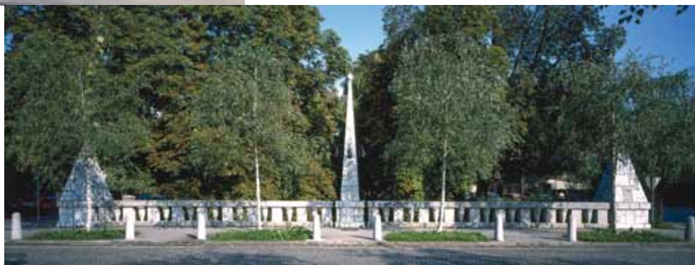
▶ Ograja mostu s piramidama in svetilko v obliki vitke piramide v sredini (foto: B. Zupančič). Bridge balustrade with two pyramids and a slender pyramid lamp in the middle (photo: B. Zupančič).
