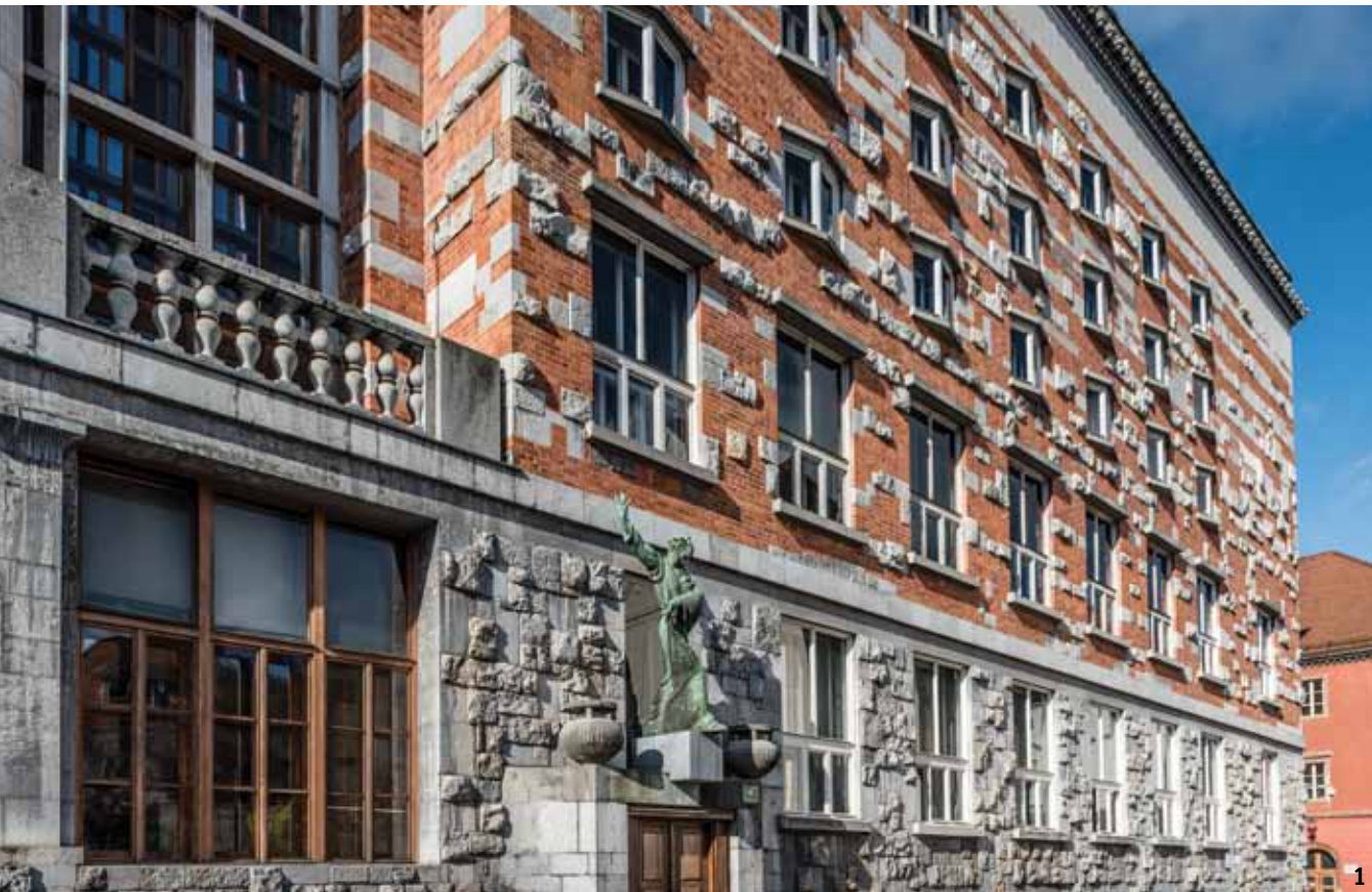
1 Narodna in univerzitetna knjižnica, detajl pročelja z okni ter menjavo kamnov in opeke (foto: B. Zupančič). National and University Library, facade detail with windows and alternating stone and brick (photo: B. Zupančič).
