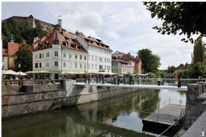
3 Most čez Ljubljanico, 2014, arh. Peter Gabrijelčič (foto: P. Gabrijelčič). Bridge across the Ljubljanica River, 2014, architect: Peter Gabrijelčič (photo: P. Gabrijelčič).
